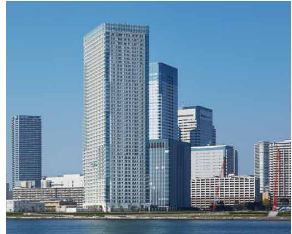
The Parkhouse Harumi Towers Chronoresidence (completed in 2013), which epitomizes our disaster-management standards
