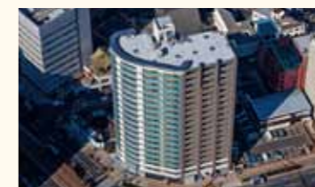
Hiroshima: The Parkhouse Hiroshima Ekimaedoori (Completed in 2013)
