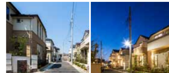
The Parkhouse STAGE Oizumi Gakuen (Completed in 2014)
