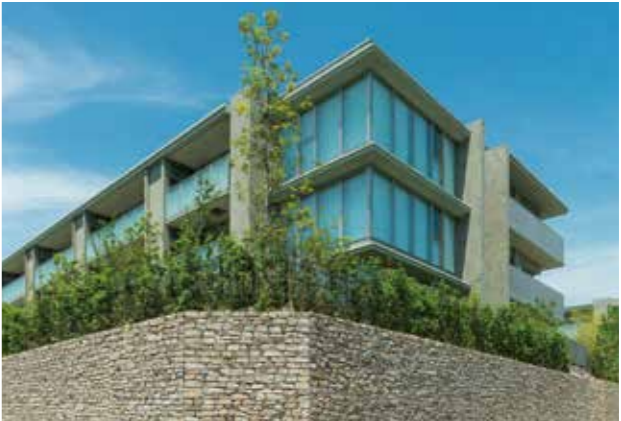
The Parkhouse Ashiya (Completed in 2015)
