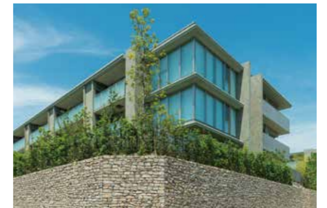
The Parkhouse Ashiya (Completed in 2015)
