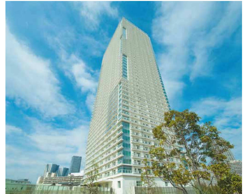
The Parkhouse Harumi Towers Chronoresidence (completed in 2013), which epitomizes our disaster-management standards
